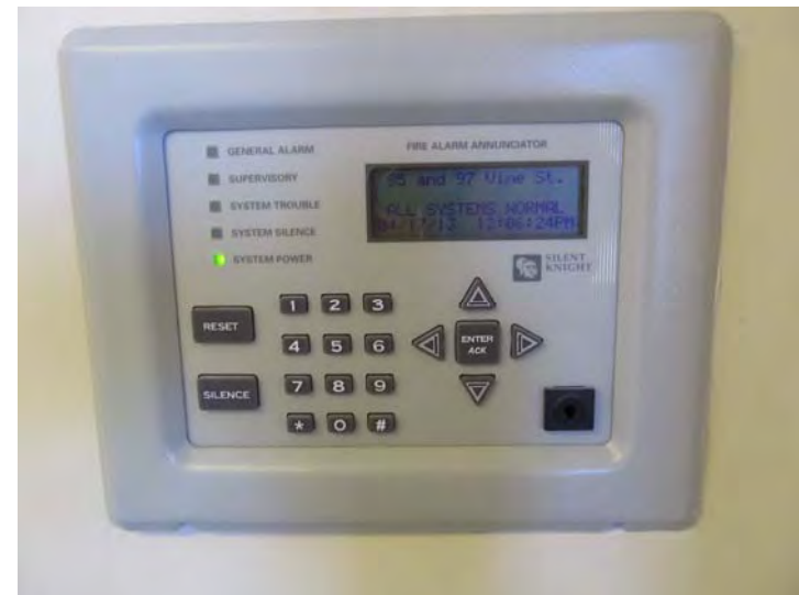
Newer, fully addressable, fire alarm control panel
