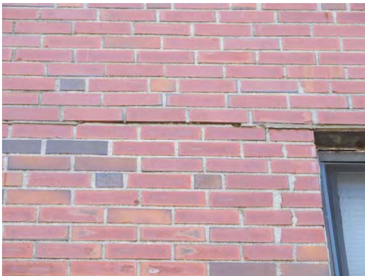
Mortar loss noted at window corners at various locations around building
