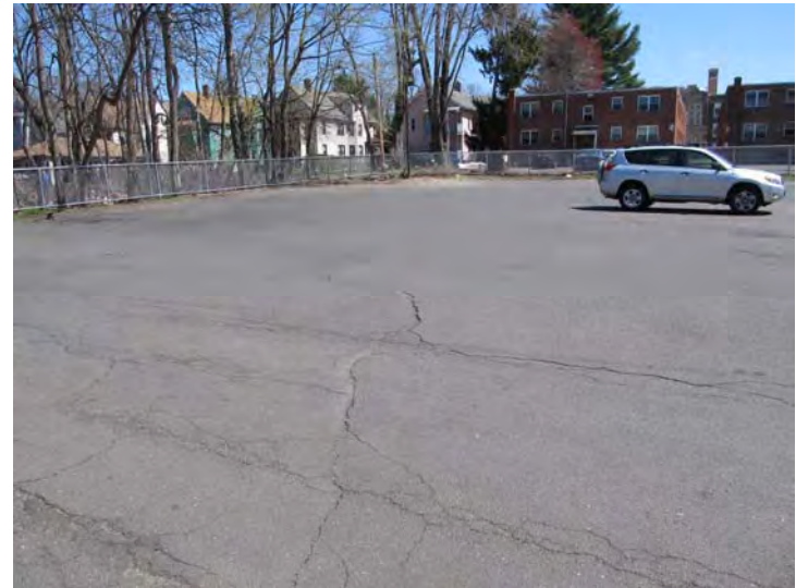
Asphalt paving exhibits some age related wear and cracks
