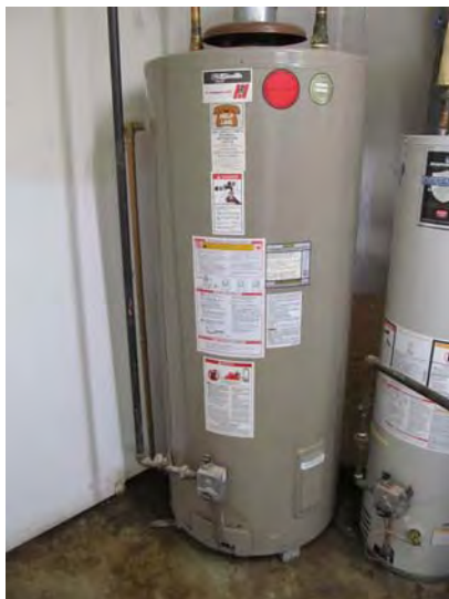
Natural gas-fired domestic hot water tank for common areas
