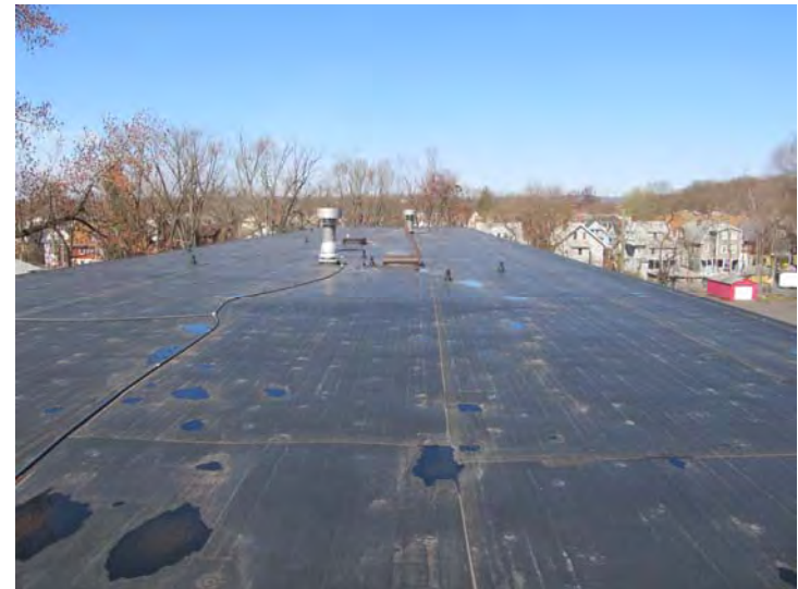
Fully adhered rubber membrane roofing system is in good overall condition
