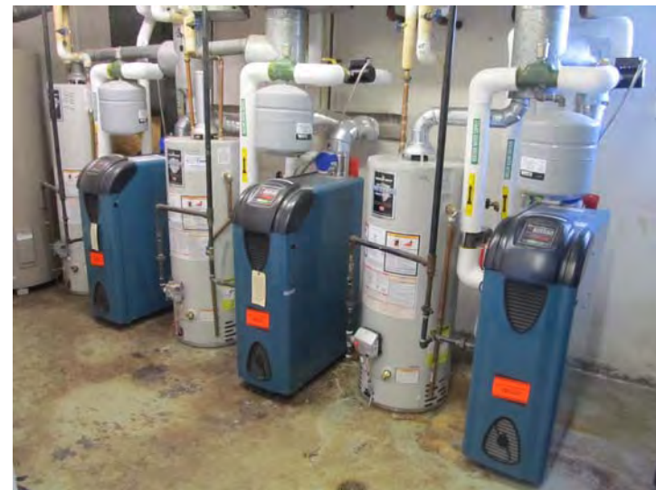
Each unit is equipped with its own natural gas-fired hydronic boiler and domestic hot water tank
