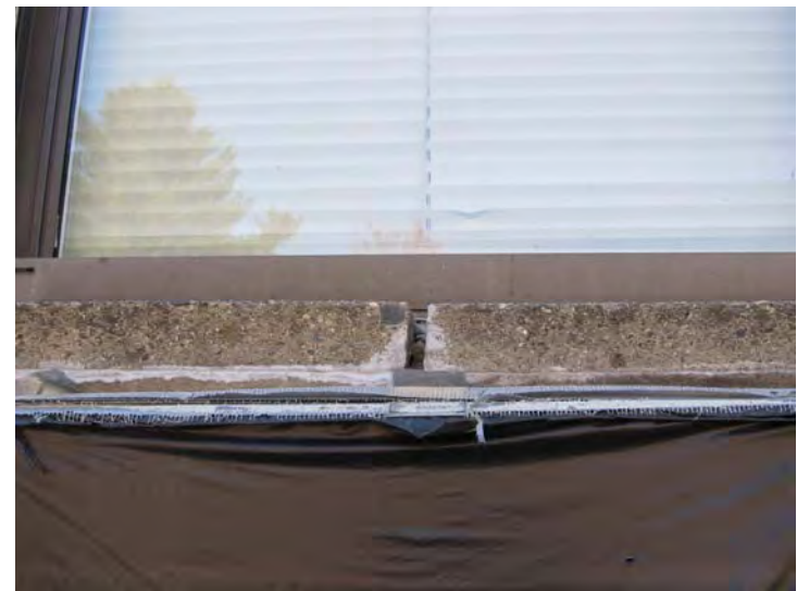
Mortar loss between concrete windowsill sections also noted at various locations
